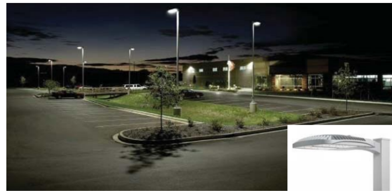
Parking Lot Lighting
